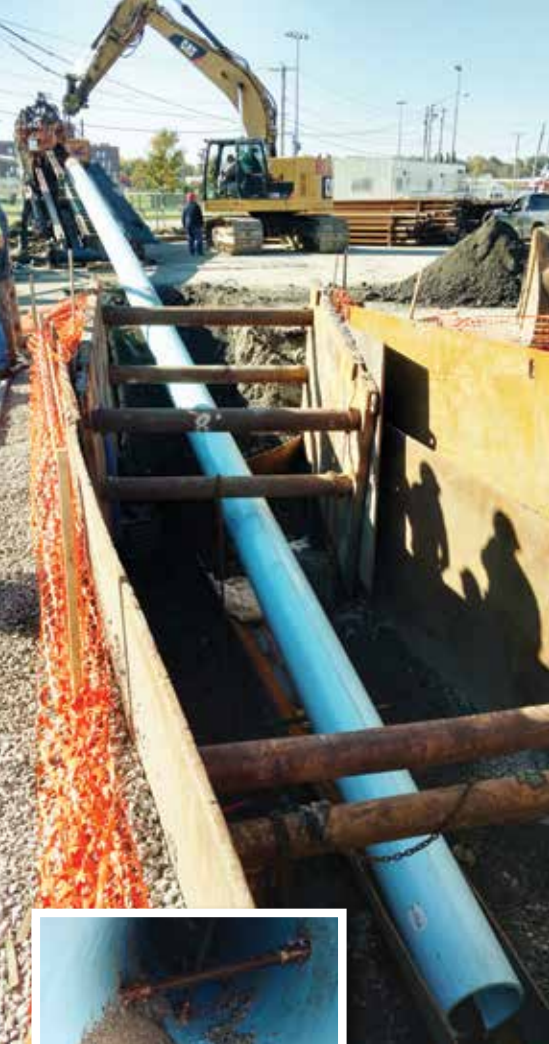
90-foot "Prover Piece" revealed an unanticipated issue as shreds of the host pipe's epoxy coating were sheared off during the pull and debris sucked into the PVC pipe
