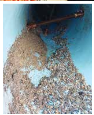
90-foot "Prover Piece" revealed an unanticipated issue as shreds of the host pipe's epoxy coating were sheared off during the pull and debris sucked into the PVC pipe
