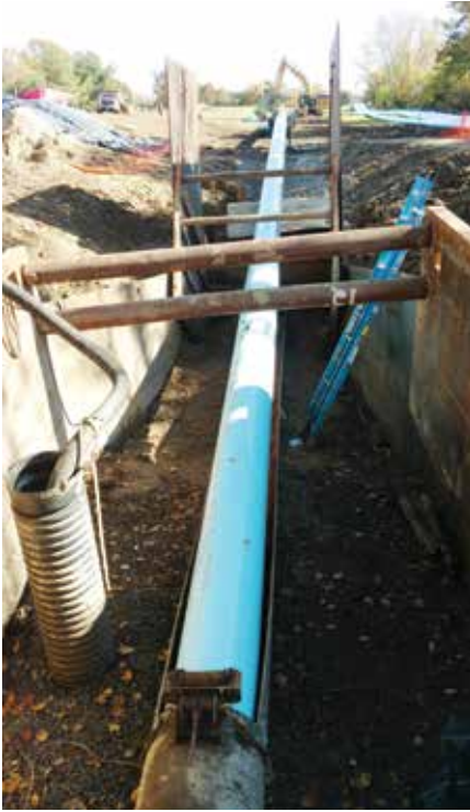
PVC pipe was pulled from the golf course side of the river to the Port of Providence side. Sliplining pull completed in 3 days
