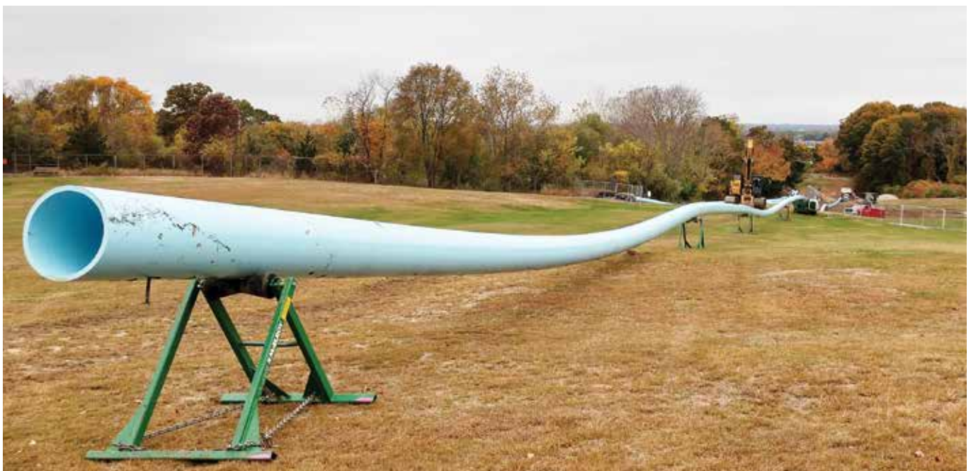
PVC was fused into 450-foot lengths, 10 sections of pipe in total
