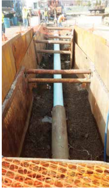
PVC pipe was pulled from the golf course side of the river to the Port of Providence side. Sliplining pull completed in 3 days
